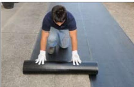
1. Unroll the second roll of modified bitumen membrane, overlapping it to the first by 10-12 cm
