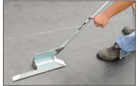
3. Start up the lap torch through piezoelectric ignition
