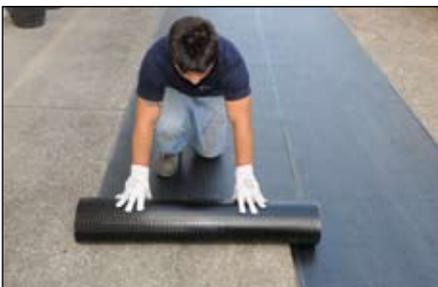
1. Unroll the second roll of modified bitumen membrane, overlapping it to the first by 10-12 cm
