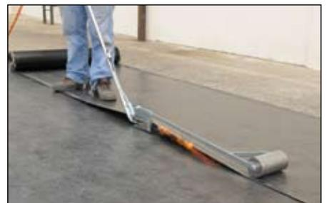
3. After starting the torch, put the lap shoe under the second membrane, heating and pulling towards oneself
