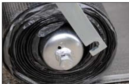
5. Hook the machine to the roller by the two forks and begin the heating of the membrane pulling the machine towards you
