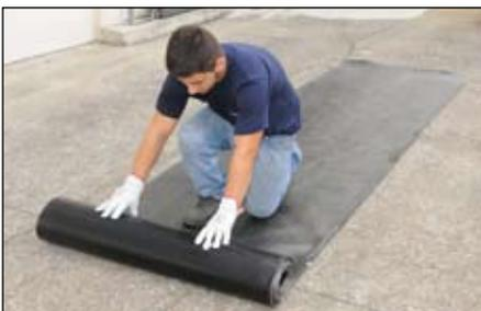
1. Unroll the modified bitumen membrane, cut it and put it straight
