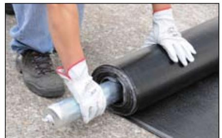
3. Insert the iron roller into the roll
