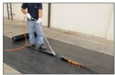
2. After starting the torch, put the lap shoe under the second membrane, heating and pulling towards oneself
