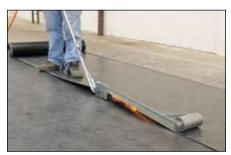
**3.** After starting the torch, put the lap shoe under the second membrane, heating and pulling towards oneself
