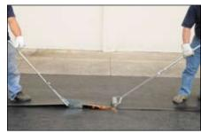
**3.** At the same time the second operator will seal the joints pressing with the roller
