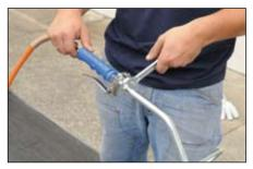
2. Tighten the lap torch nut with a 22 mm spanner
