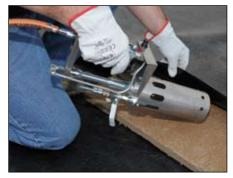
**3.** The hot air roofing burner reduces the danger of open flames and can be used on different kinds of surface.
