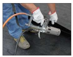
**3.** Light the hot air roofing burner by pressing the piezoelectric ignition. Pull the lever and turn the head towards the surface to be heated, keeping it at a distance of about 20 cm
