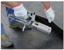
2. Pull the lever and turn the head towards the surface to be heated, keeping it at a distance of about 20 cm
