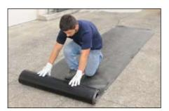
**1.** Unroll the modified bitumen membrane, cut it and put it straight
