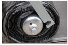
**5.** Hook the machine to the roller by the two forks and begin the heating of the membrane pulling the machine towards you
