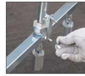
**4.** Fix the safety bracket with the wing nuts
